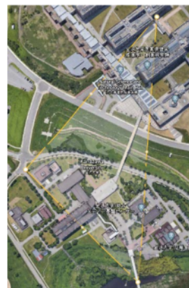
Fig. 14. ES920LR LoRa Test on Building and Trees Obstacles.
