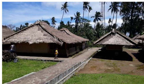
Fig. 6. The use of pavement on pedestrian lines is expected to have an impact on the site and the originality of the traditional village Sasak Senaru.
