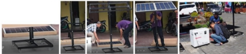
Figure 8: Installation of Portable Bracket & Photovoltaic Energy Solar Panel (20 minutes)
