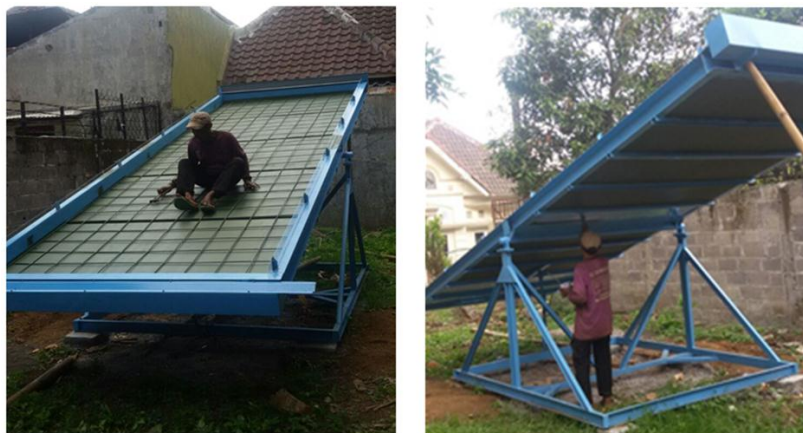
Figure 5. Installation of sloping plot of paving blocks.
