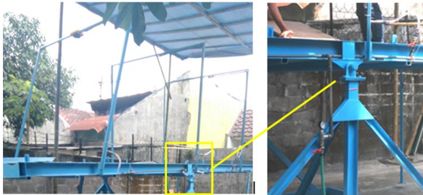
Figure 6. Installation of rainfall simulator on the sloping plot
