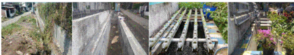
Figure 2. Transformation of the study site, starting before the drainage channel improvement project, the construction phase, modification of the channel for fish and vegetable cultivation.
