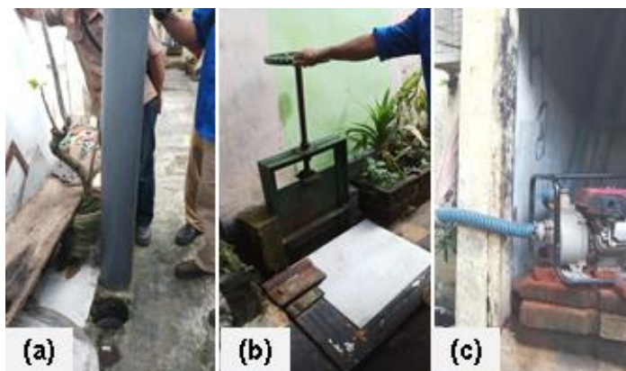
Figure 3. The existing flood resilience system consists of water level indicators at subsurface sewer (a), sluice gates for controlling water level (b), and pumping stations to raise water to the nearest receiving water body (c)
