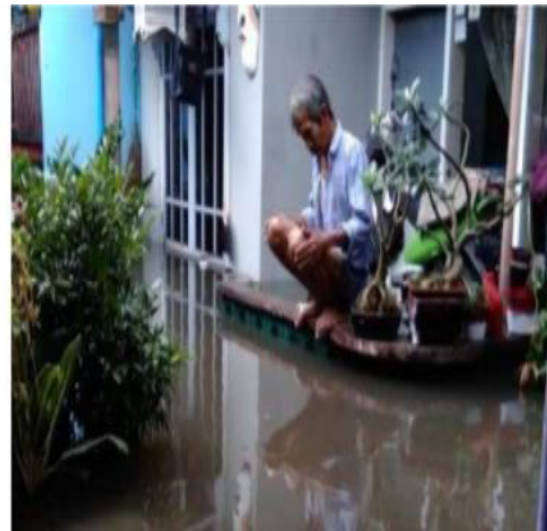
Figure 2: Inundation conditions in residents' houses RW 05 Purwantoro Village
