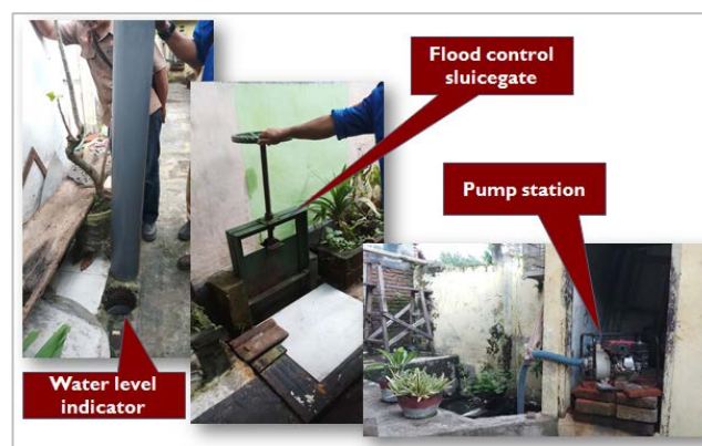
Fig. 2. Simple flood resilience structure; source: own elaboration
