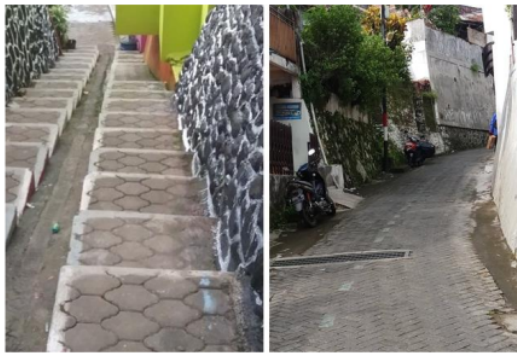
Photo 6. Paving block on sloped surfaces in the study area (phot. L. Sedyowati)
