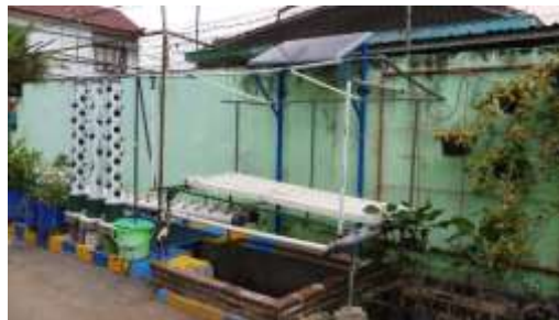
Photo 3. The installation of solar cell to supply energy for circulating water from the drainage channel
