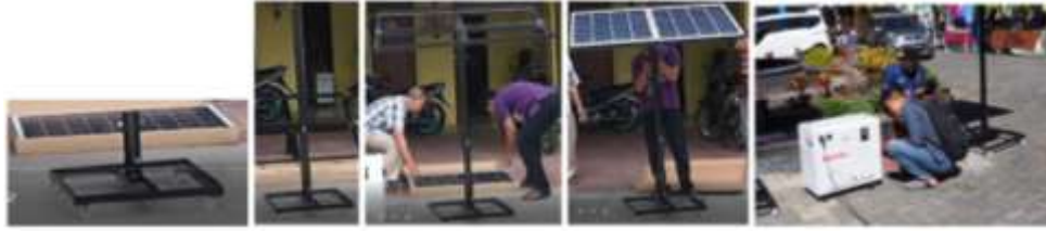
Figure 11: Installation of Portable Bracket and Solar Photovoltaic Energy Panels (20 min)
