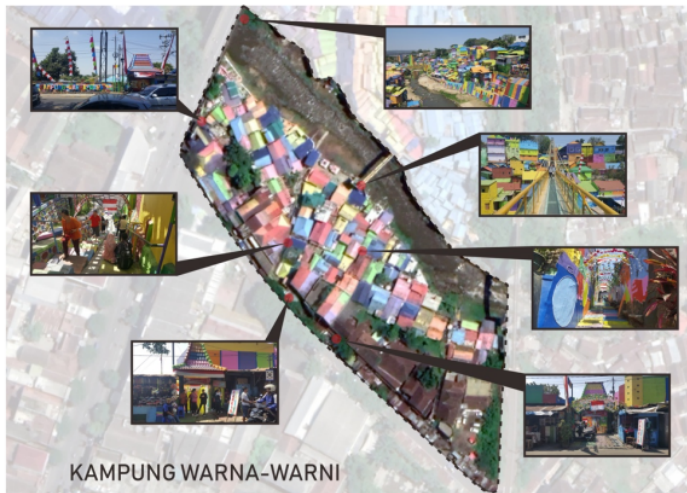
Figure 3. Aerial view of Kampong Warna-warni Jodipan, Malang city
