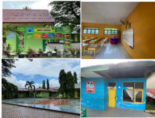
Figure 2. The condition of SMPN 1 Darul Imanah Source: Author documentation (2023)
