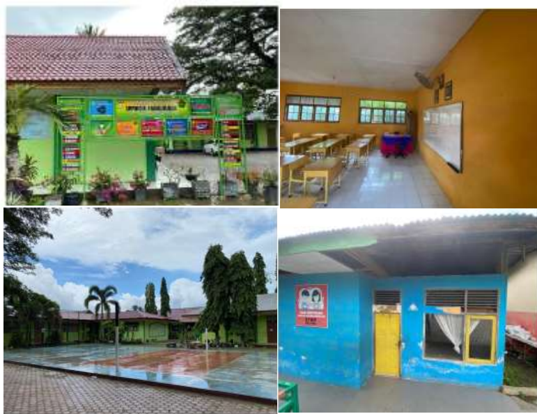
Figure 2. The condition of SMPN 1 Darul Imanah
