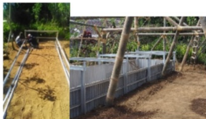
Figure 5. Hydrogamic Installation (6 days)
