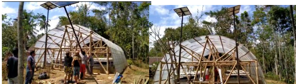
Figure 6: PLTS Installation (2 days)
