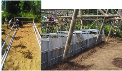
Figure 5. Hydroganic Installation (6 days)
