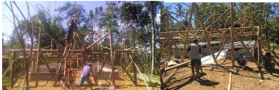
Figure 4. Construction of a Greenhouse (15 days)
