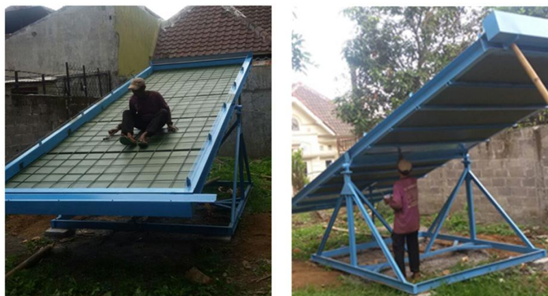
Figure 5. Installation of sloping plot of paving blocks.
