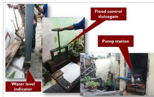
Fig. 2. Simple flood resilience structure; source: own elaboration
