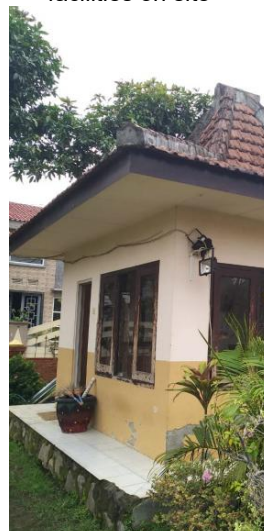
Figure 7. Toilet and security office
